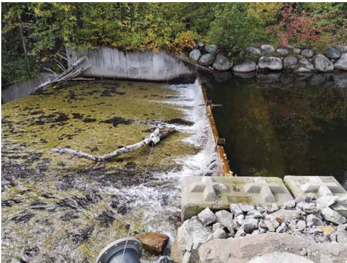
Figure 4-7 Trepanier Creek Reach 3 Stop Logs Observed on September 27, 2019.
