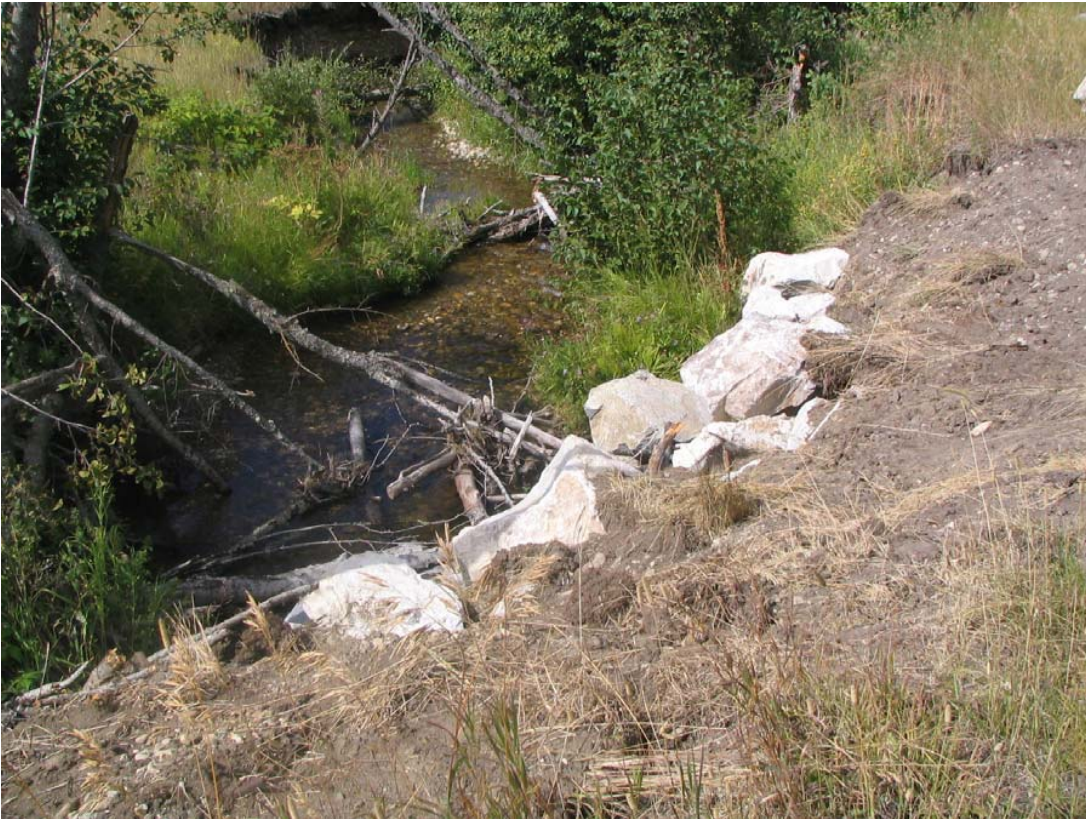
Photo Plate 7: Rip rap stabilization of stream bank.
