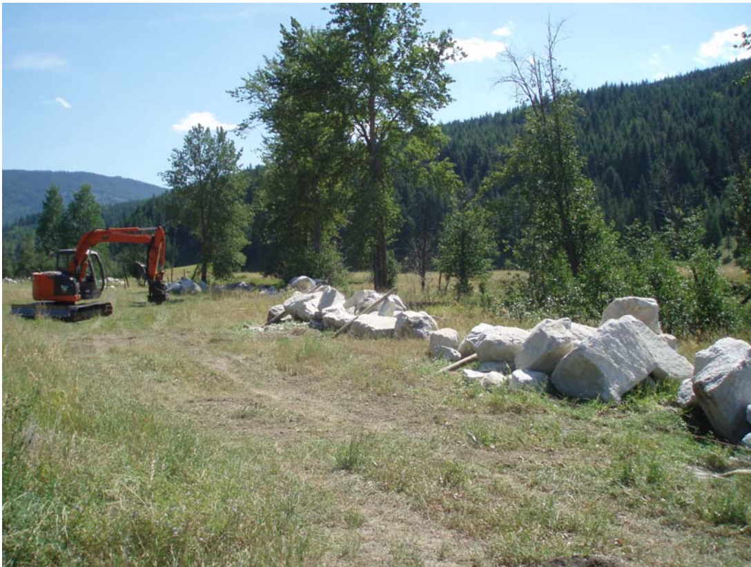
Photo Plate 3: Rip Rap Rock to be installed in channel.
