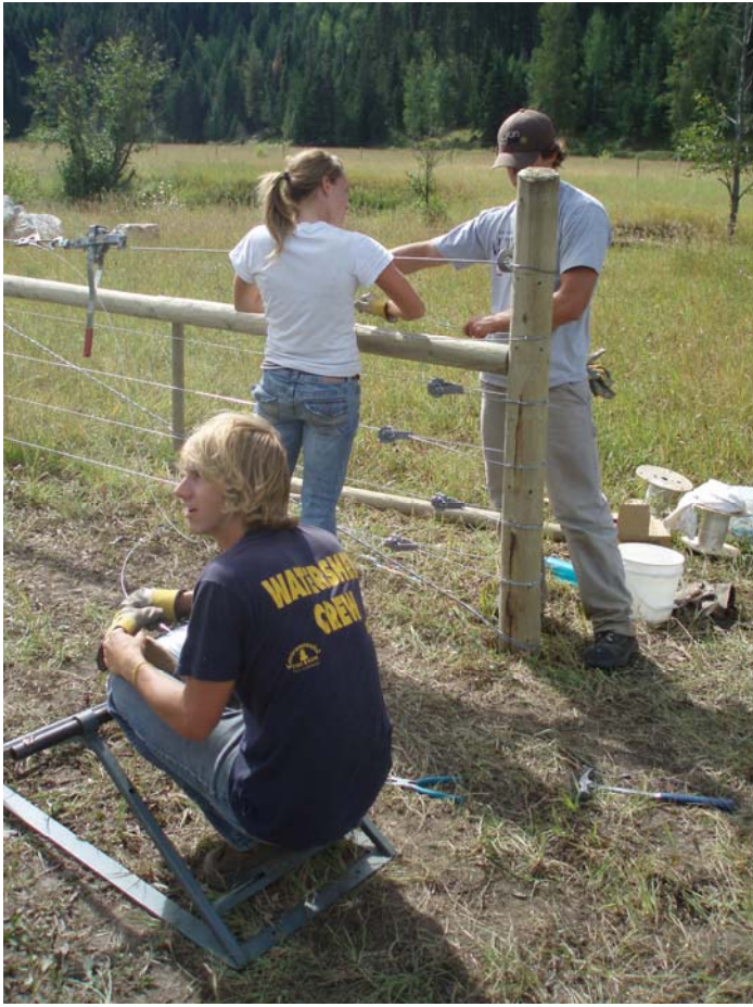
Photo Plate 10: Installation of fencing by joint RDCO / City of Kelowna watershed restoration crew.
