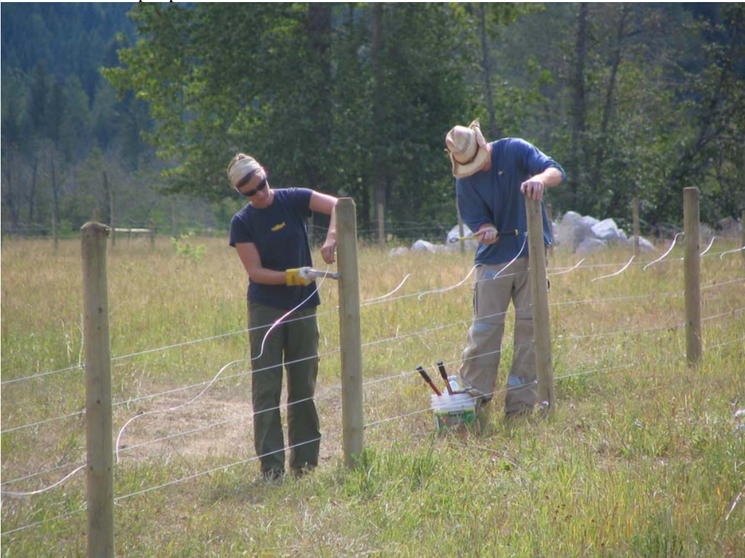
Photo Plate 9: Installation of 6 strand high tensile wire.
