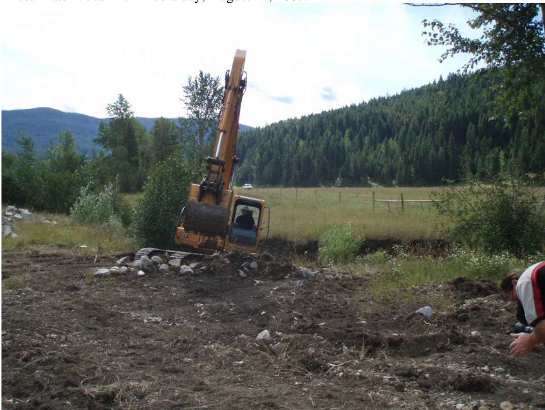
Photo Plate 2: In-stream work including installation of rock structures.
