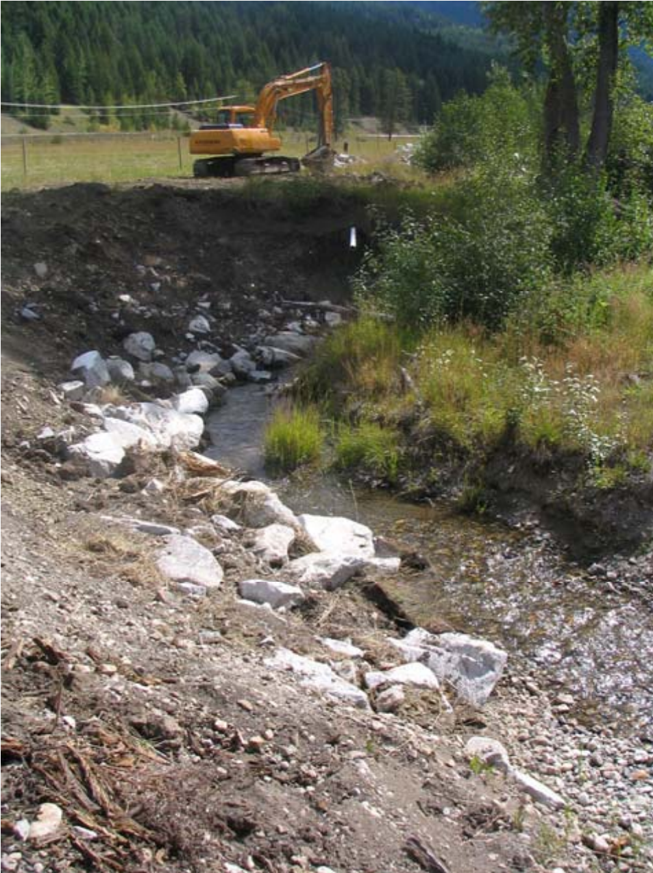
Photo Plate 11: Larger eroding bank stabilization prior to grass seeding and planting.
