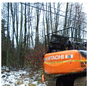
Backhoe set on fire and drilling rig window smashed
