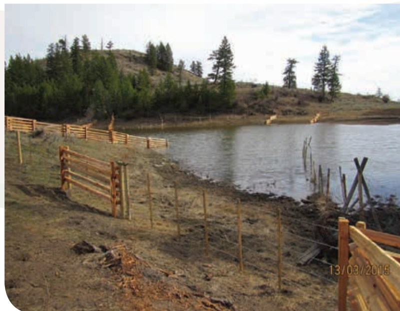
Photo: Stink Lake wetland fencing, Courtesy Jillian Tamblin
