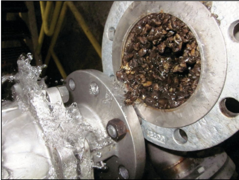
Here is what a water intake pipe looks like with invasive mussels.
