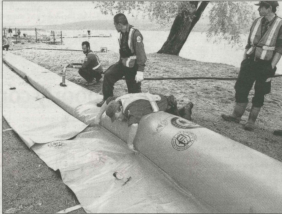
Crews install a bladder dam at Pritchard Park in West Kelowna last spring to combat flooding concerns. Photo: Alistair Water/Capital News
