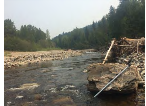
2 Replaced hydrometric station on Mission Creek - upper reach.
