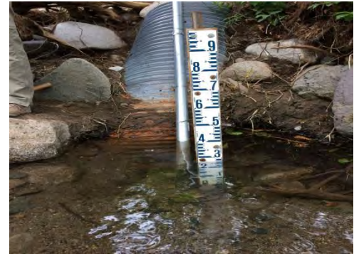
1 Replaced hydrometric station on Shorts Creek
