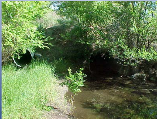
Culvert (5' dia.) at ~ RM 0.20 (looking upstream)
