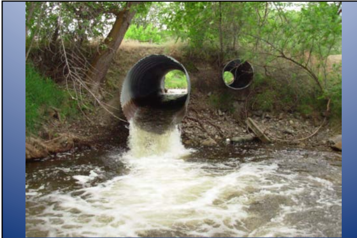
Culvert at Burdett Street (~ RM 0.1)
