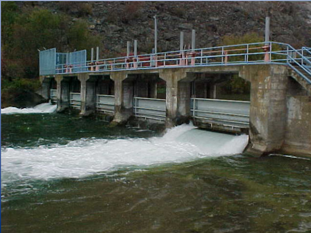
McIntyre Dam – Oliver, British Columbia
