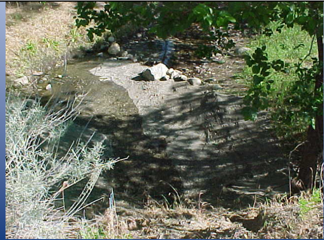
Culvert (5' dia.) at ~ RM 0.25 (looking upstream)
