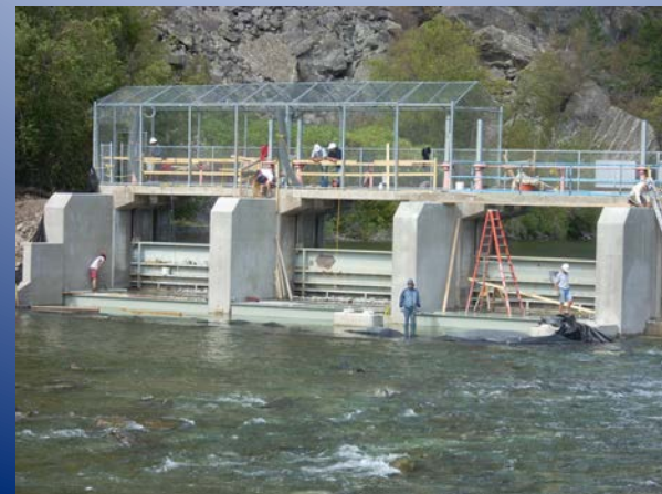
McIntyre Dam – September 2009
