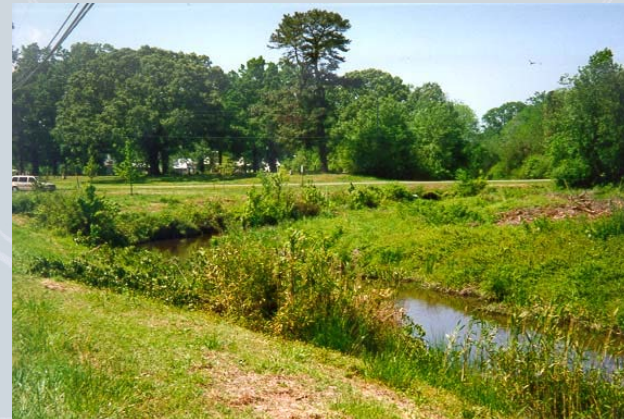
Ditch that flooded, carried polluted water
