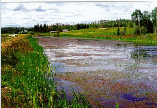
Prince George, BC Constructed Wetland
