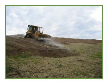
Biosolids are used in landfill closures. Biosolids-based "biocovers" treat methane produced by landfills reducing GHG emissions.
