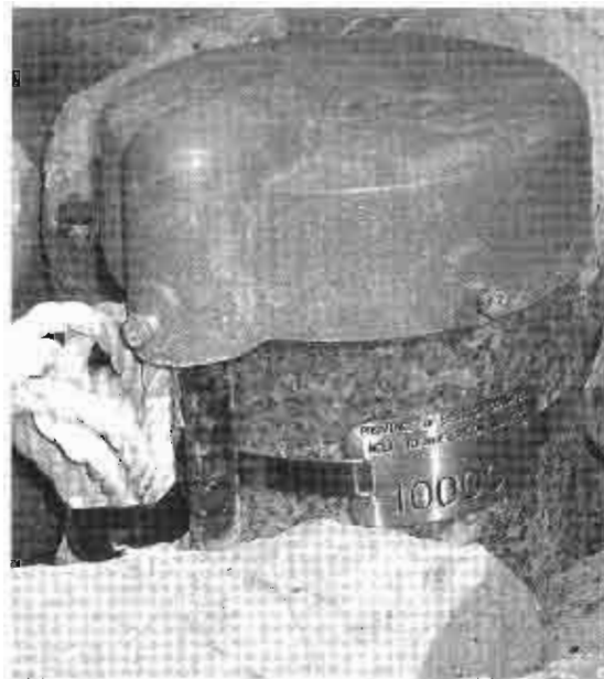
Well identification plate attached to a well.
