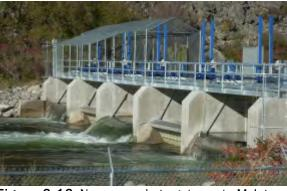
Figure 2.13: New overshot gates at McIntyre Dam to enable fish passage.
