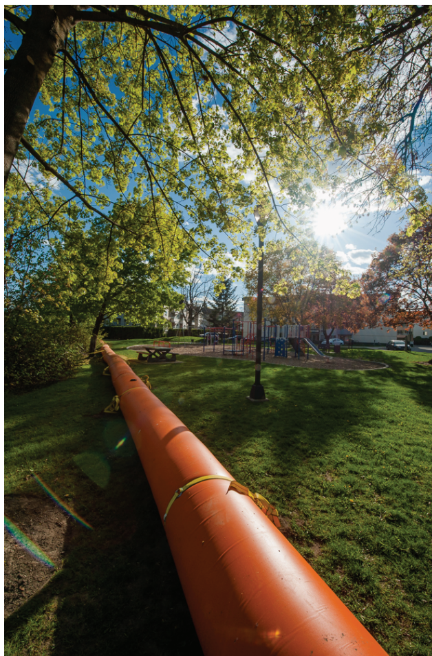
Inset 6-1 Temporary flood barrier in the City of Kelowna, photo courtesy of City of Kelowna - Michael Hintringer
