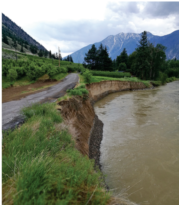
Inset 6-2 Erosion resulting from the 2018 freshet, photo courtesy of the RDOS.
