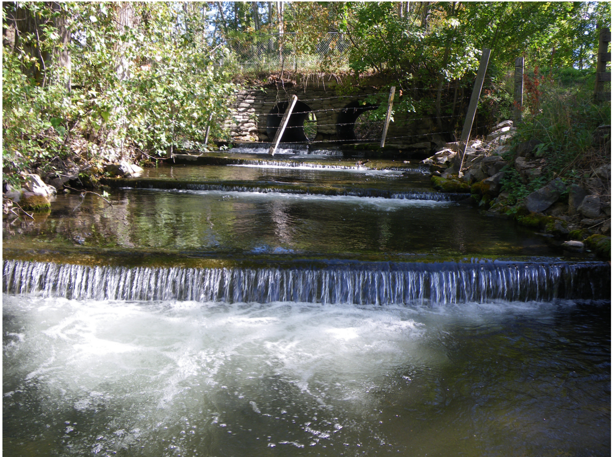
Photo 3: Culvert crossing with enhancements downstream (i.e. constructed weirs and associated scour pools)
