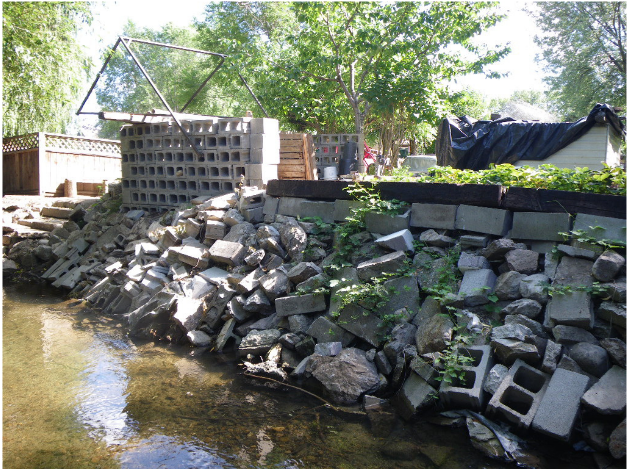
Photo 2: Bank armoring in a modified residential area along Coldstream Creek
