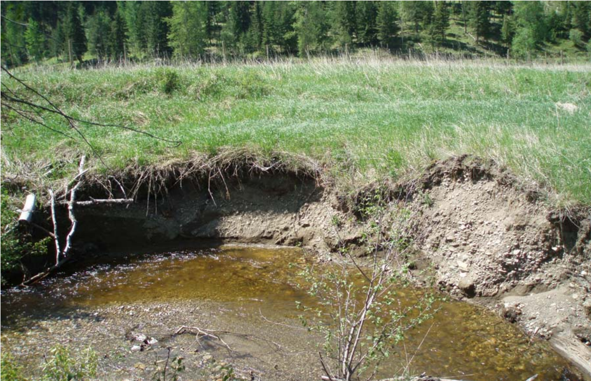
Photo Plate 6: Additional eroding bank due to upstream failure of riffle structure. This site has been identified as a priority for maintenance and enhancement.
