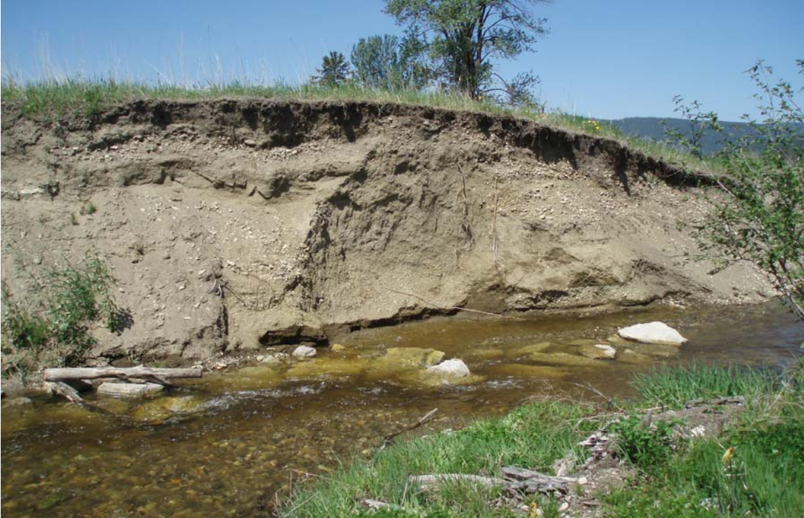
Photo Plate 5: Failed bank stabilization flagged as a priority for maintenance and enhancement. June 2, 2009.
