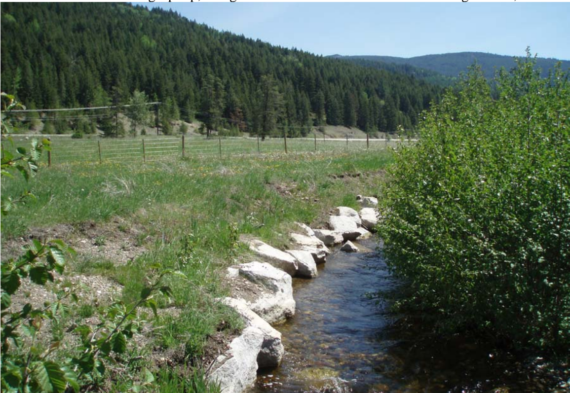
Photo Plate 2: Functioning rip rap, revegetated bank and cattle exclusion fencing. June 2, 2009
