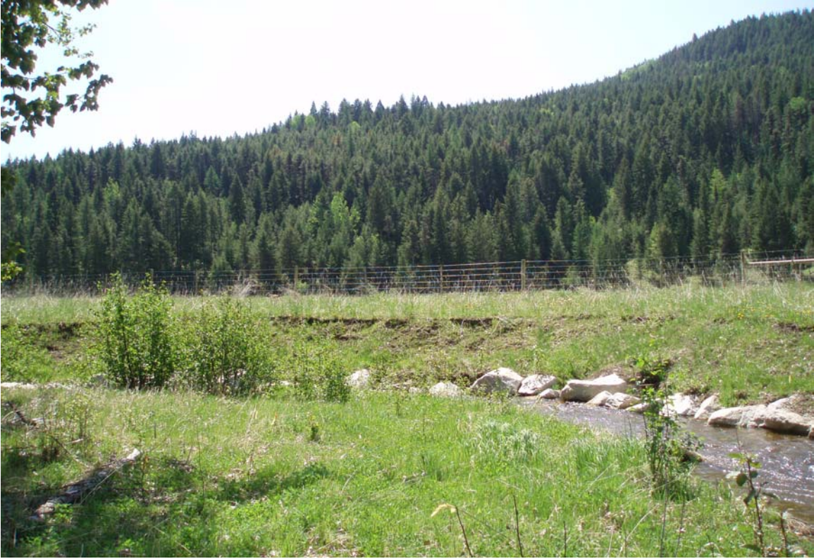
Photo Plate 1: Functioning rip rap, revegetated bank and cattle exclusion fencing. June 2, 2009.
