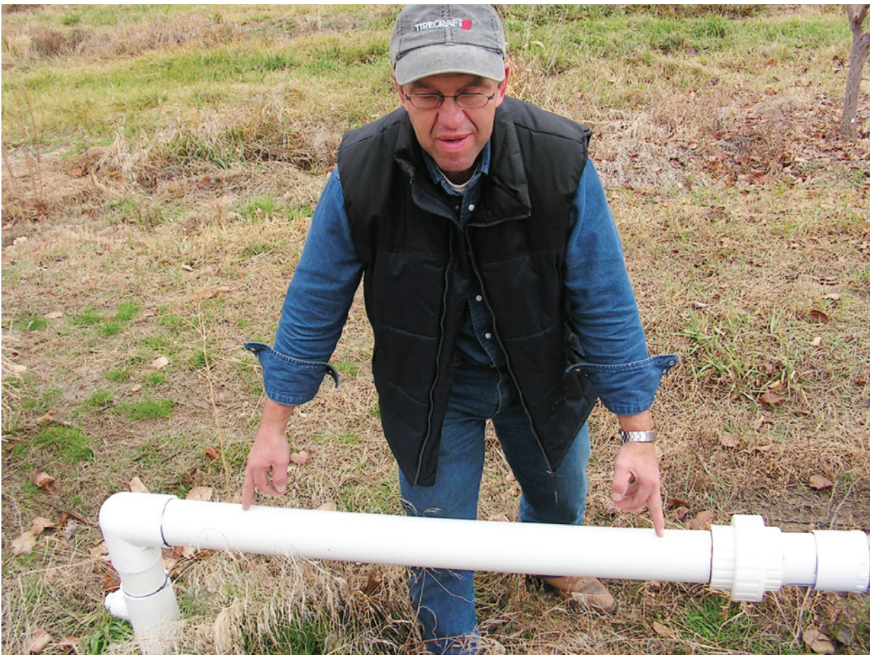
Bill Stewart indicates the portion of the new above ground valve structures designed for the installation of water meters in the future.
