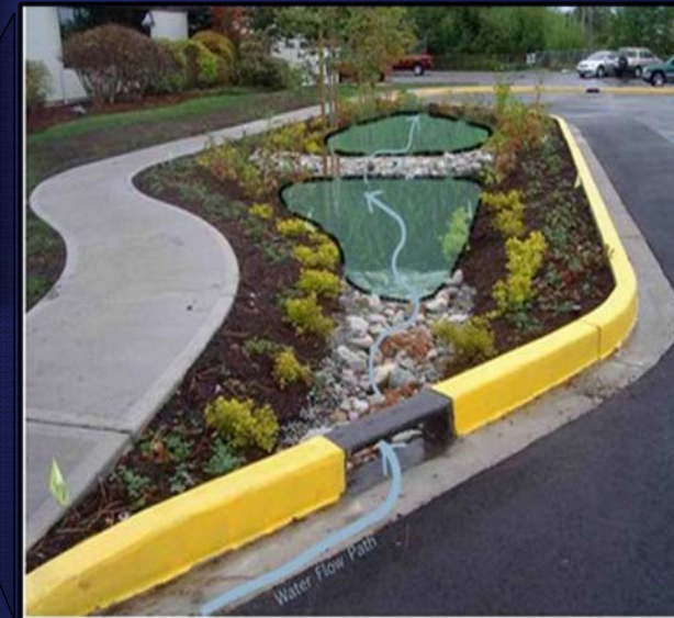
Trent St Rain Garden
