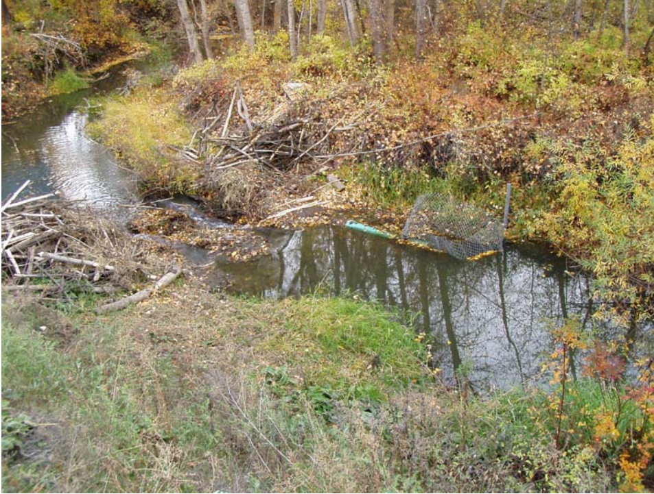
Photo 1. The beaver dam by the “God Sign” was modified to allow additional passage of water. Small channels were also formed on the top of the beaver dam to facilitate fish passage.
