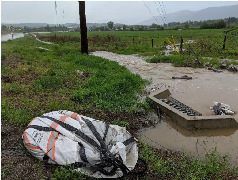
Figure 1-4: Emergency culvert blockage north of Rosedale Rd E & Hwy 97A - May 9, 2018 (looking north)
