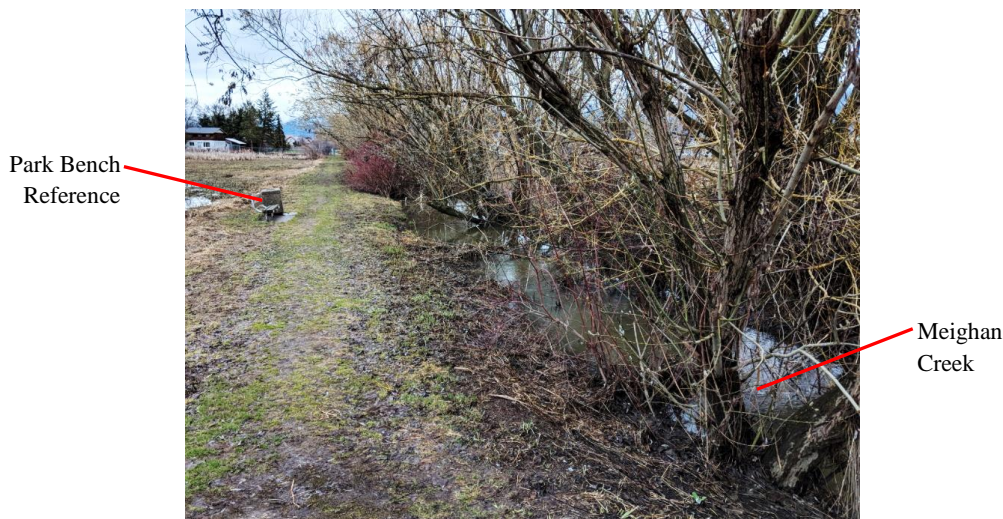
Figure 2-16: Sediment deposition and heavy vegetation growth in thalweg just upstream of Okanagan Road on Meighan – low flow conditions (April 7, 2018)
