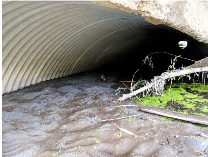
Figure 2-17: Sediment deposition in culvert – Wood Avenue right culvert shown
