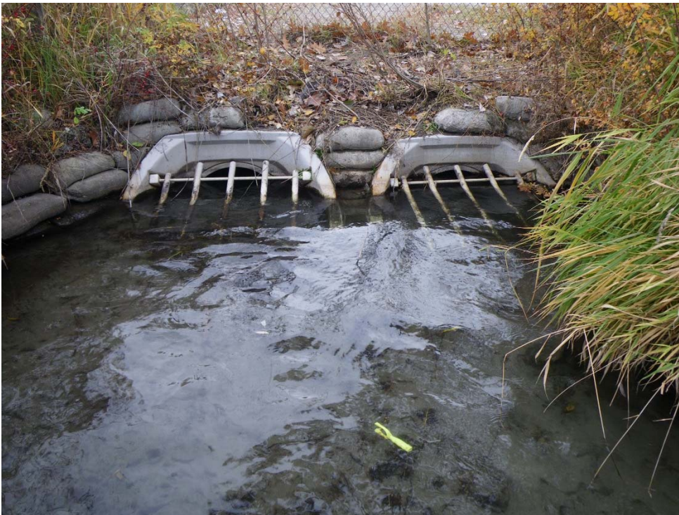
Photograph 4: Downstream end of culverts (November 2009). Credit: Ecoscape
