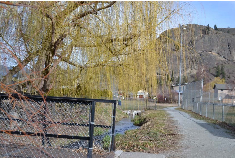
Photograph 6: Looking downstream at bridge crossing from Dale Park to Prior Place (11 March 2016).
