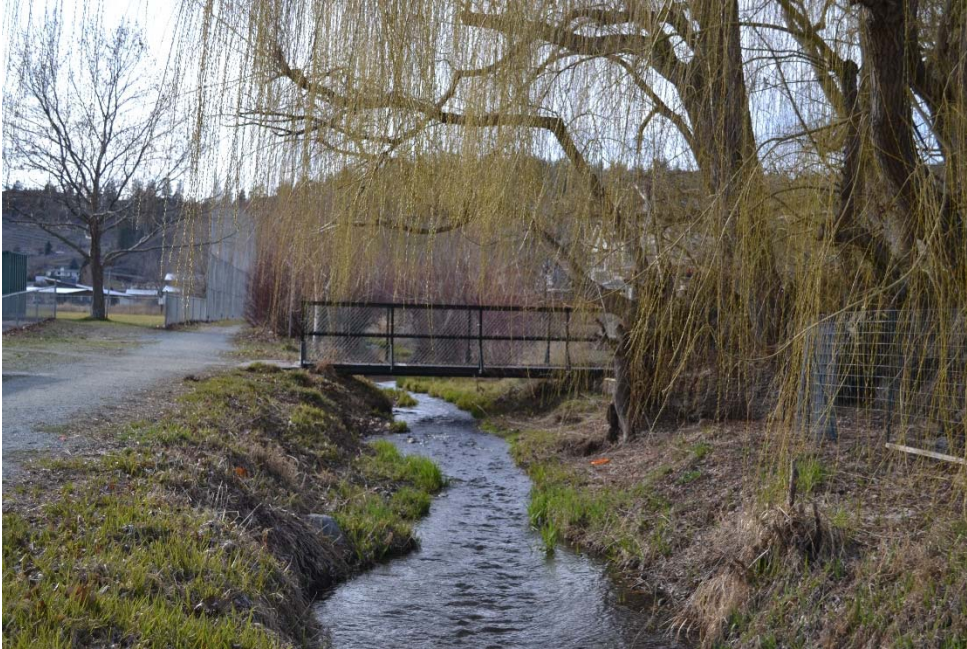
Photograph 5: Looking upstream at Prairie Creek from culverts at Giants Head School ground (11 March 2016).
