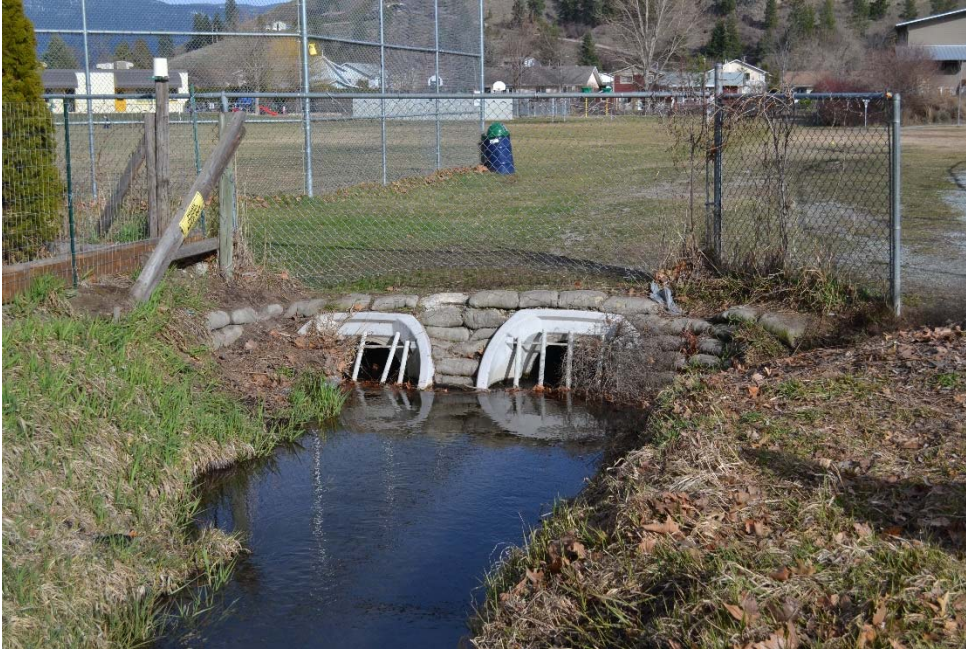
Photograph 3: Upstream end of culverts (11 March 2016).
