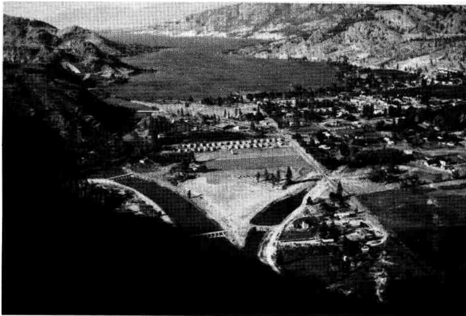
Photo 2 OKANAGAN FLOOD CONTROL CANAL AND SHUTTLEWORTH DEBRIS BASIN - D.S. #16 (in foreground) Flow 300 c.f.s. - Looking North (Sept. 12, 1973)
