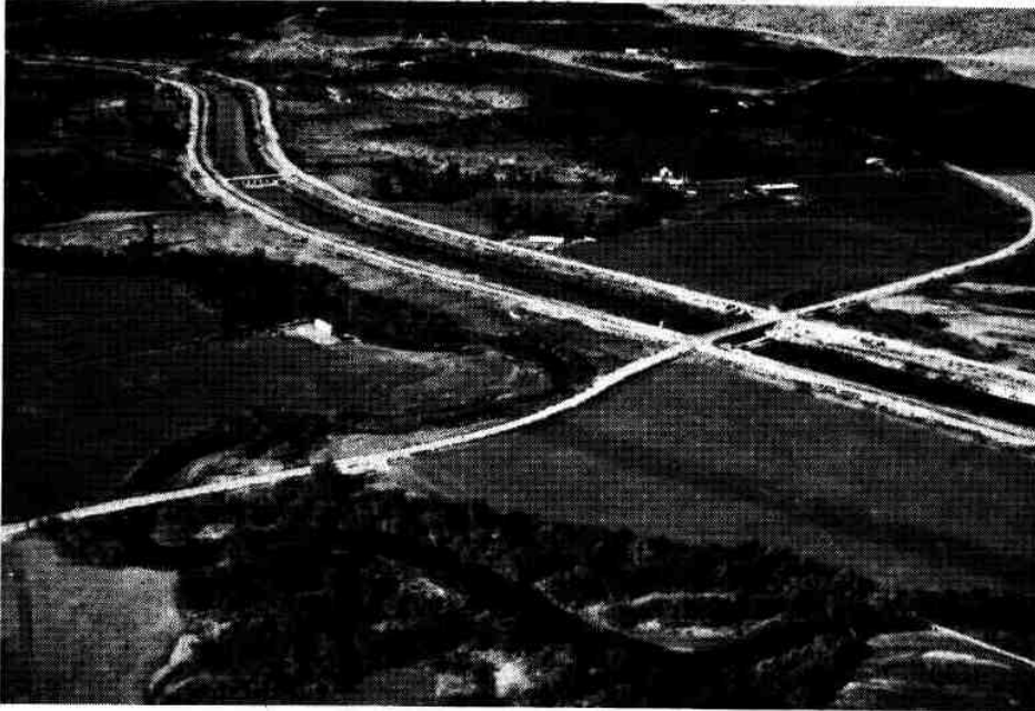
Photo 9 OKANAGAN FLOOD CONTROL CANAL showing Oxbows D.S. #3 (in foreground) - Flow 300 c.f.s. Looking North (Sept. 12, 1973)
