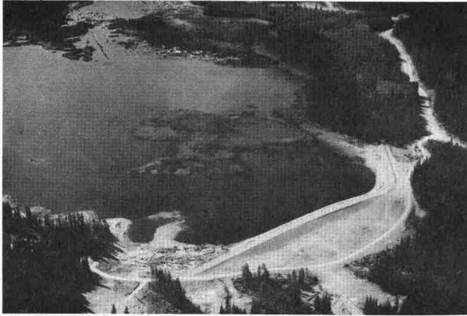
Photo 35 LAMBLY LAKE showing North Dam Looking Northeast (Sept. 12, 1973) Powers Creek System
