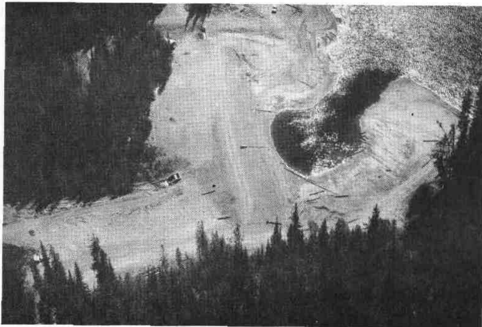
Photo 34 JACKPINE LAKE DAM Showing details of control works Looking Southwest (Sept. 12, 1973) Powers Creek System
