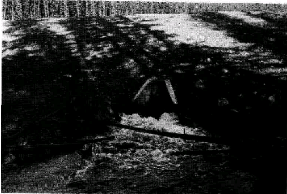
P hoto 16.5 Earth dam, west end of Crooked Lake with discharge outlet
