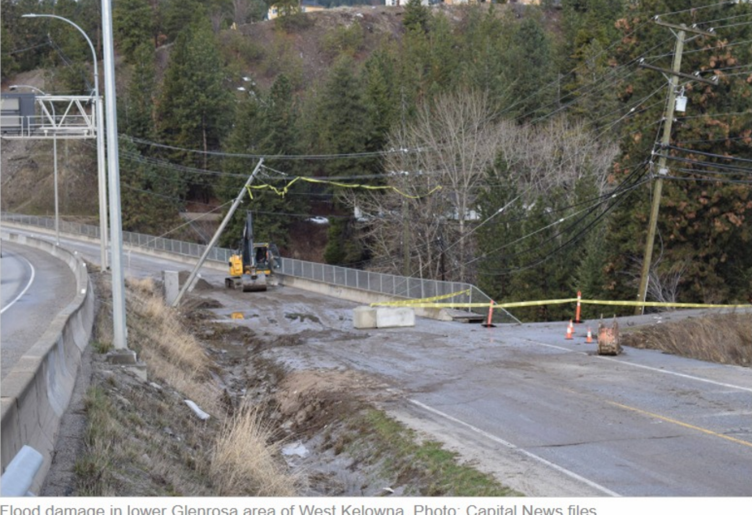
Flood damage in lower Glenrosa area of West Kelowna. Photo: Capital News files
