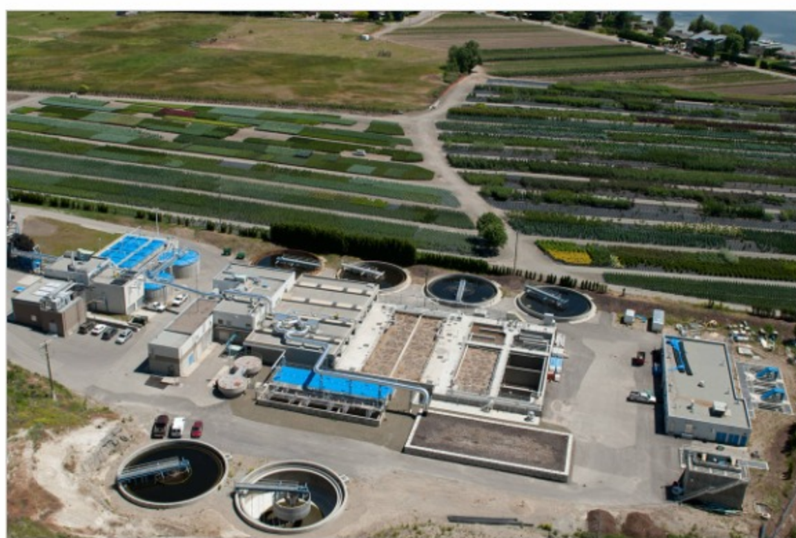
Each day, the plant located off Gellatly Road in West Kelowna treats an average of 10 million litres of wastewater. —Image: CORD
