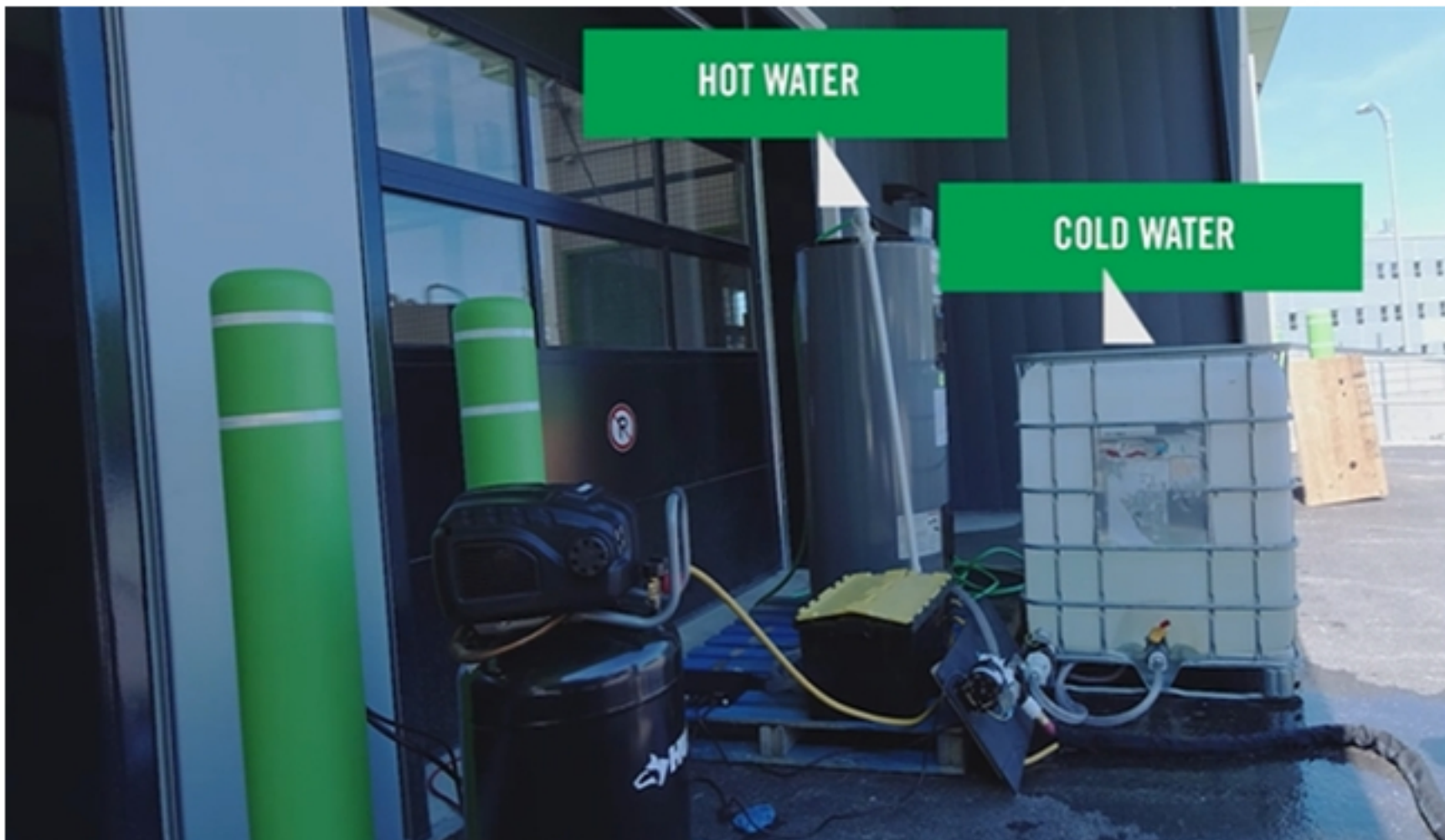
Hot and cold water is pumped into the ballast to kill the zebra mussel larvae. Image Credit: Submitted/Ozero
