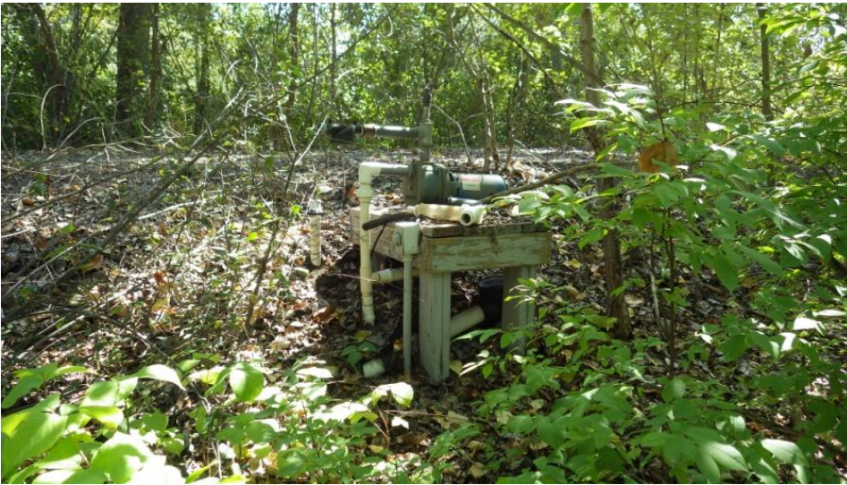
Intake #5452, no known license, pump and pipes visible but not operational at time of observation
