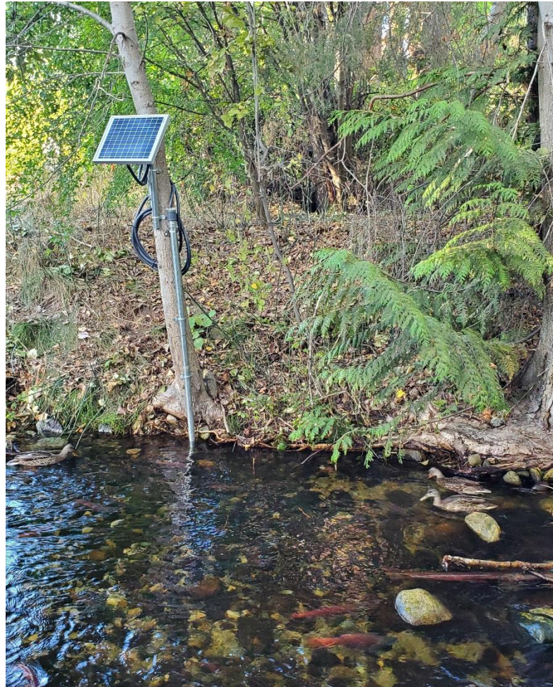
Newly installed Naramata Creek hydrometric station. Note the spawning Kokanee in the foreground.
