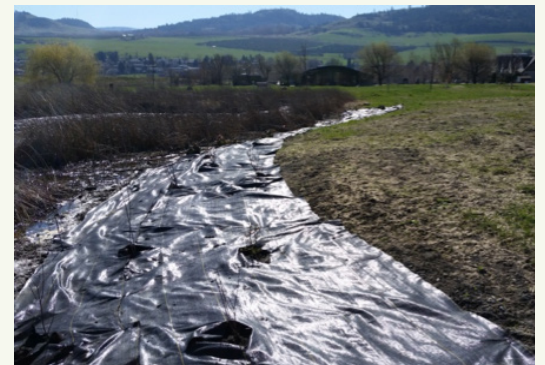
Native shrub planting adjacent to a wetland. Landscape fabric controls aggressive quackgrass. Frisbee golf course is to the right which may be removed once native vegetation is established.
