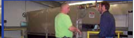
4 x 10 Rotary Drum Thickener
