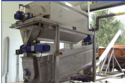
DSP Screw Press Model 3012, NY WWTP
